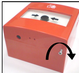
Picture 9B - locking screw installation
